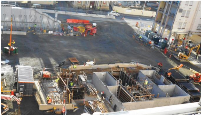
The K-Block core – lift and stairwells under construction.
