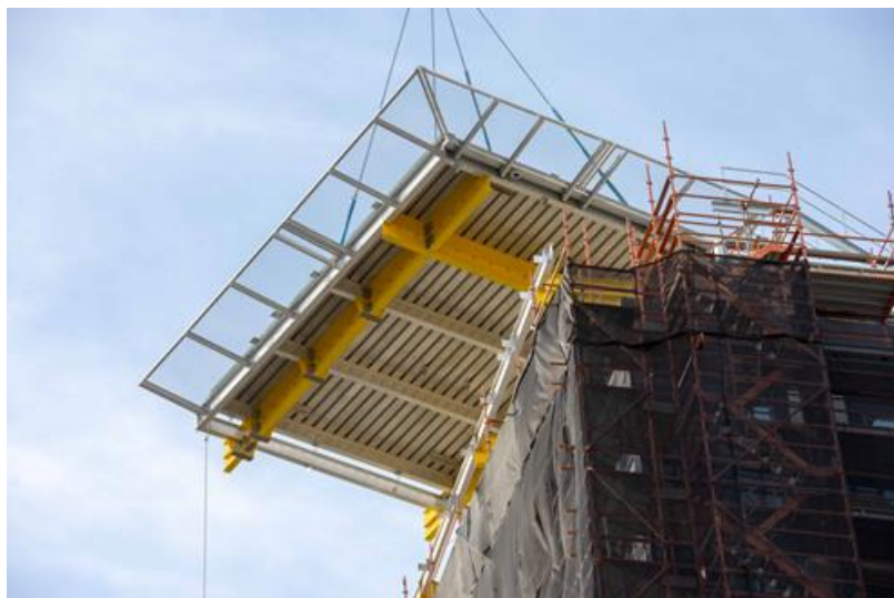
Helipad installation, 10 November 2018
