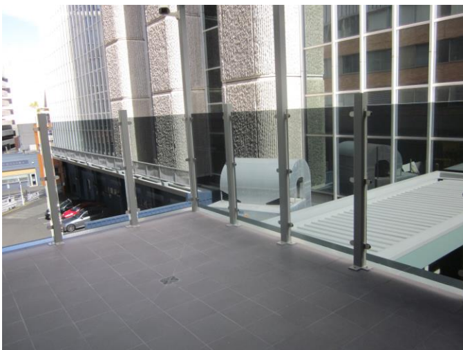
Outdoor bed bay area where intensive care patients can experience natural light and air constructed under phase 1 of the RHH Redevelopment project.
